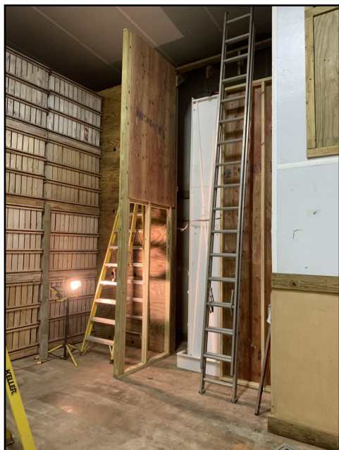
Above: Humidicell Installation. Photo: Alex Crockford.
