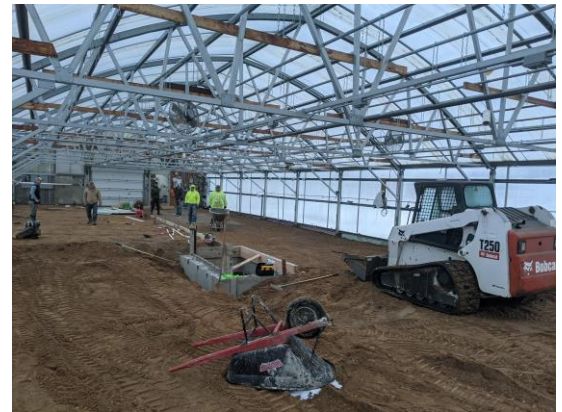
Pea Gravel floor was upgraded to concrete.
